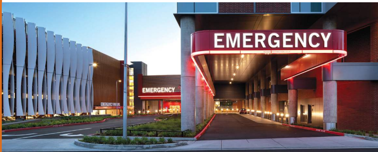
Turner Construction built Salem Hospital’s Building A expansion and Emergency Department entrance improvements.
